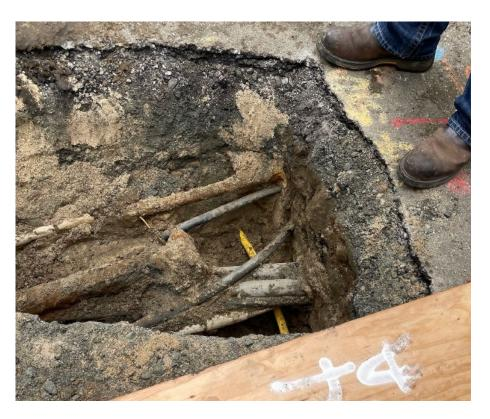
76. Another example is "Hole 15A" where the gas and electric lines were measured as being only 3.5 inches apart, as seen in the following photo:
